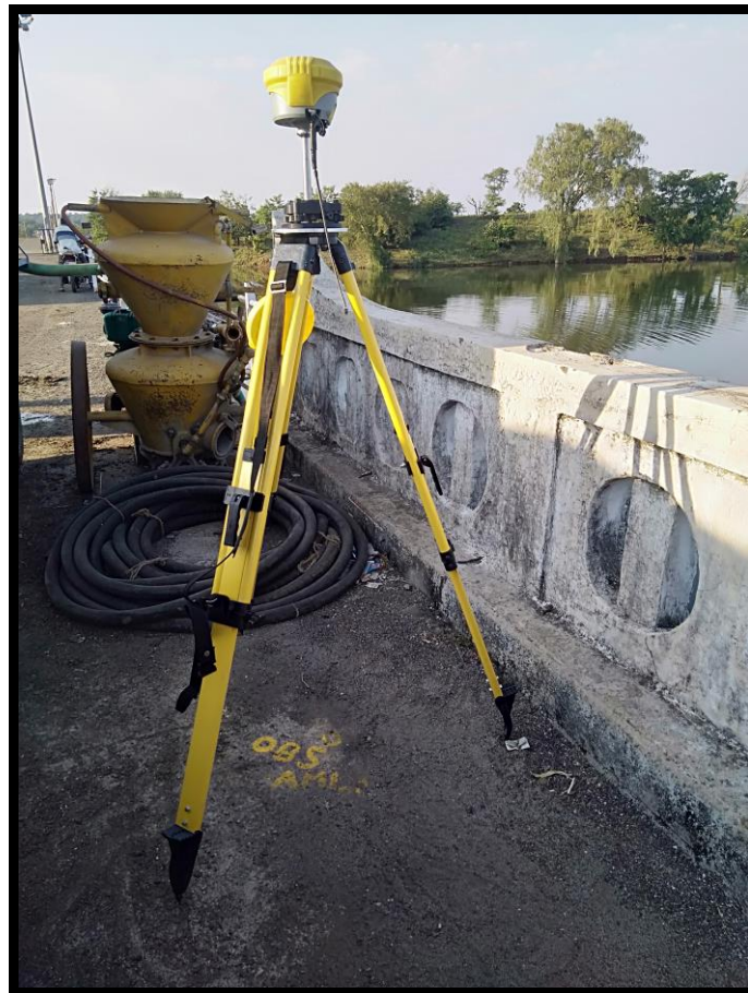
Figure 5.3-1 DGPS Observation at Dam top
